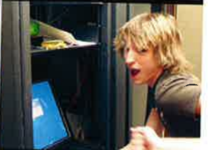
CJ Werner works in the NPHS computer server room.
