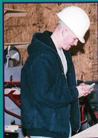
JT Francies works really hard on remodeling a house.
