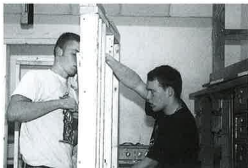
Ryan Sillery and Mike Cope do some electrical work in their Construction class.
