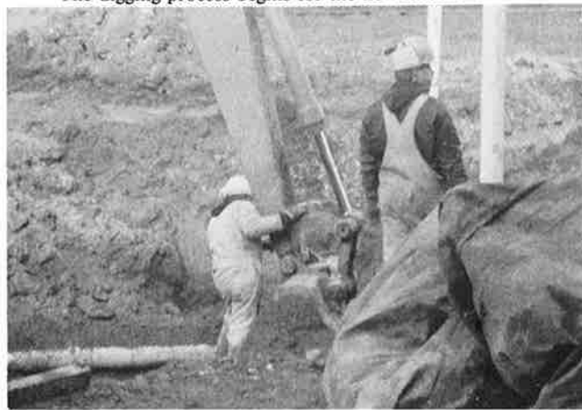
Old pipe is a pain for these workers.
