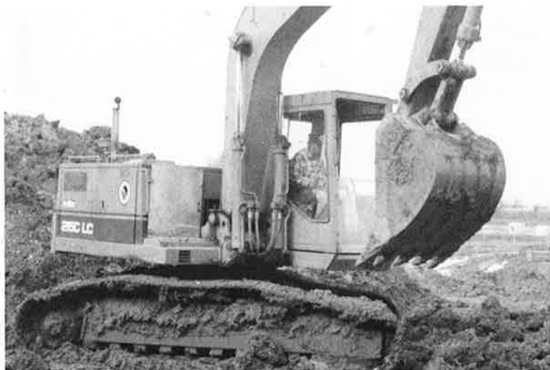
The digging process begins for the new middle school.
